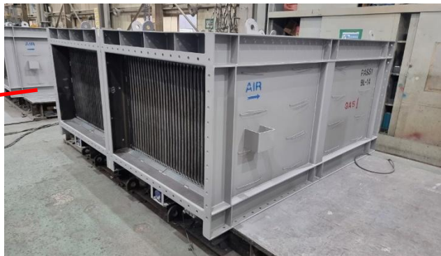
Cold APH 3 passes (Pass 1 shown) DC-01
