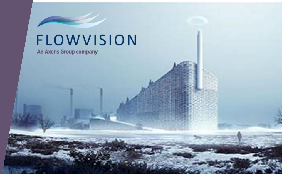
Amager Ressource Center, WtE plant. DeNOx supplied by Flowvision
